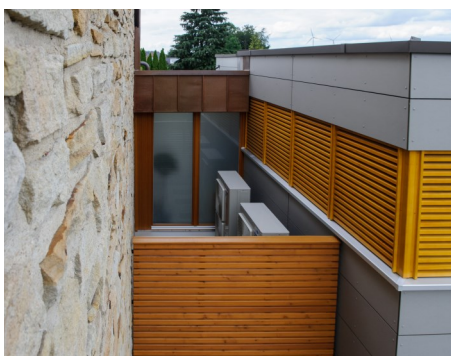
The compact outdoor Mini-ZEAS and Mini-VRV units were installed out of sight between the Chapel and new extension building.
